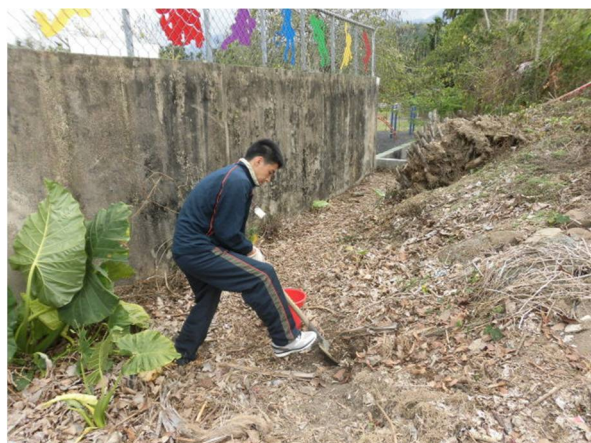
挖掘落葉腐植土
